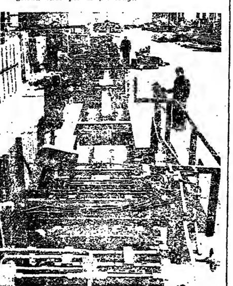
Coiled strip is fed into the underground storage loop (centre) and pulled out by a double punch roll to pass into the forming mill
